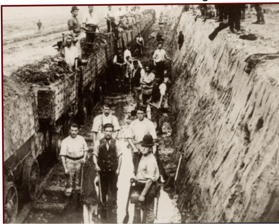
Above: Navvies working on building a canal
