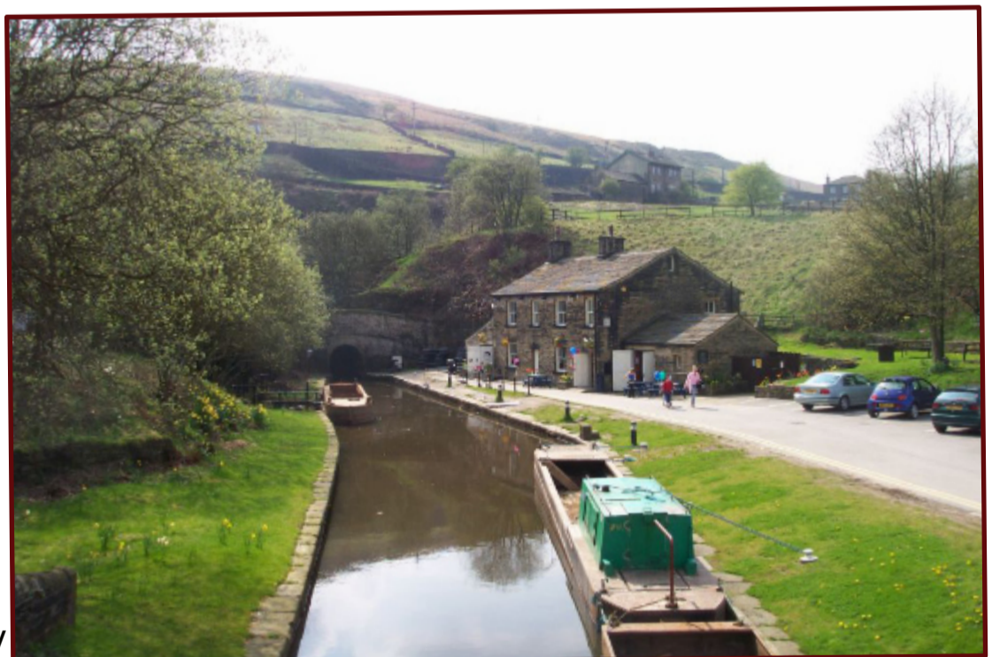
Above: Standedge Tunnel Entrance Marsden, West Yorkshire
