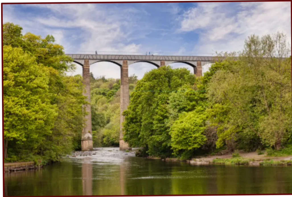
Above: The Pontcysyllte Viaduct.
