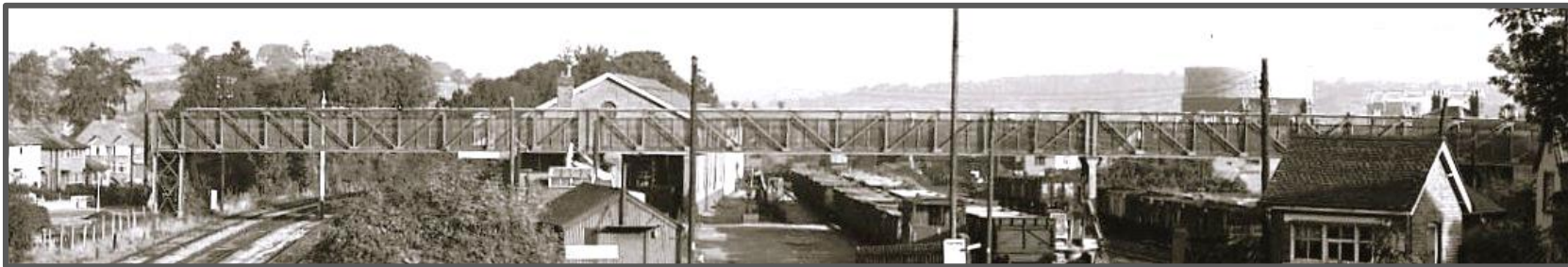
Left: The metal footbridge over the railway line and the railway which ran from Bridge Street to opposite the bottom of Bates Hill,
